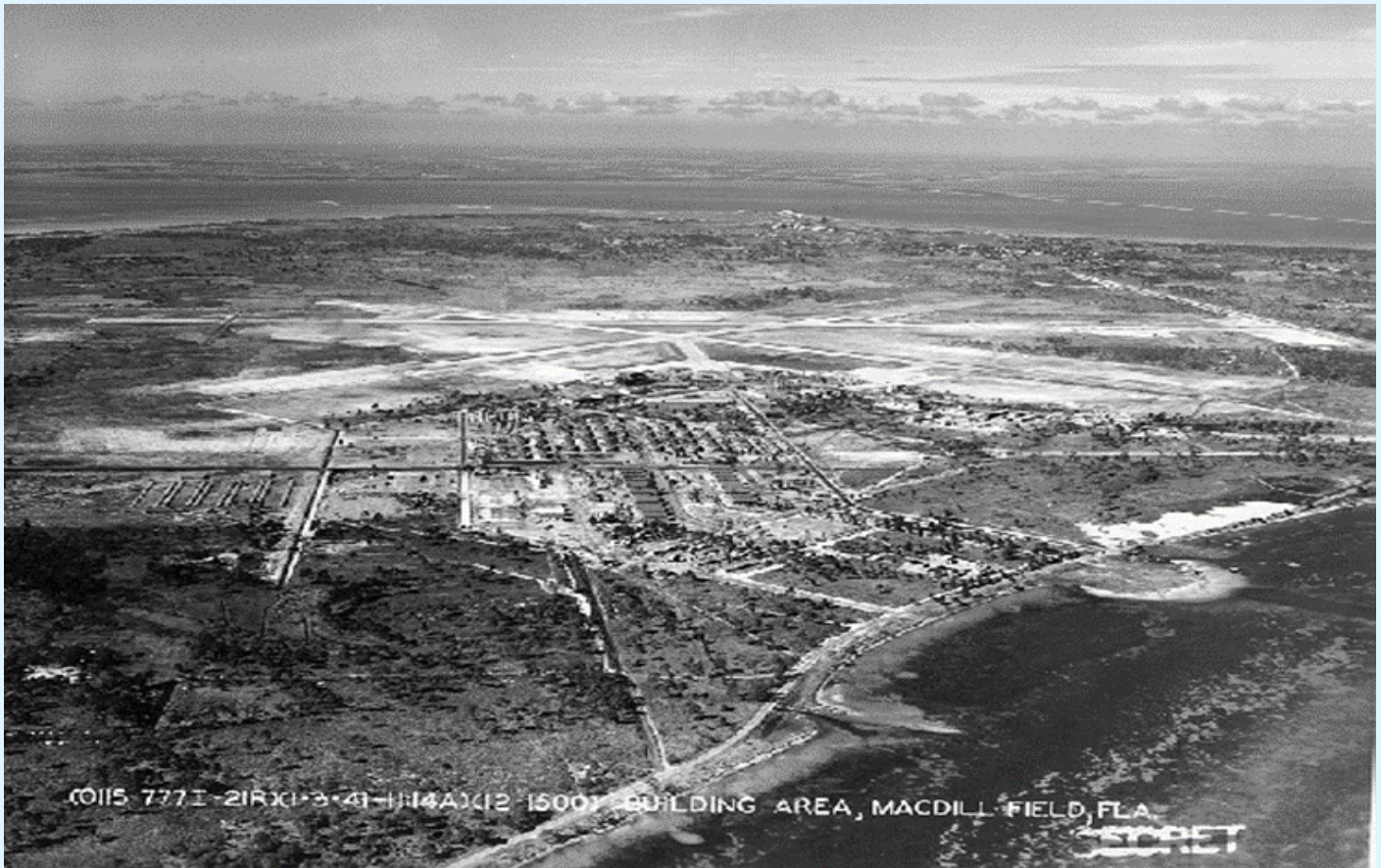
Photo Above: Southeast Air Base, Tampa (MacDill Field) under construction, June 1939
