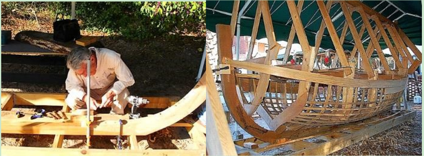
Photos Above: Heritage Boat Builder Dr. Jim Gaskins lays the keel on the strongback. The Yawl takes shape at the Museum Boat Works. Note the keel that's sitting on the strongback and forms extending down from above. This was the first of two 1760 British Yawl boats built on the Museum grounds.
